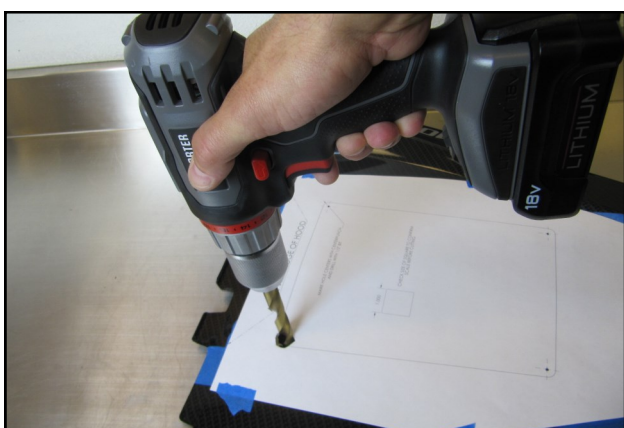
22. Using a 1/8" bit, drill out four pilot holes in the hood followed by a 1/2" bit to finish.
