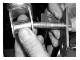
2. Connect the second "L" bracket to the other side and secure it with the 10mm Lock Nut. Note: Keep bolts loosely fasten, until the 6x45 hex bolt is inserted.
