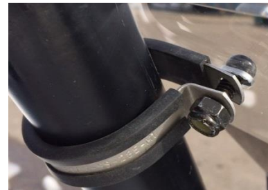
Image #2 Clamp installation detail
